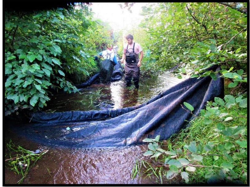
*SAB Field Supervisor Tony Meade and Field Technician Luke Chaisson installing a silt boom to catch any disturbed sediment travelling downstream during excavation.*
