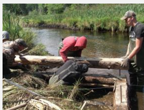
Securing the gabion logs
