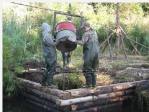
Unloading the rocks into the gabion
