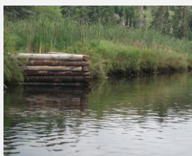
The completed gabion at North Lake
